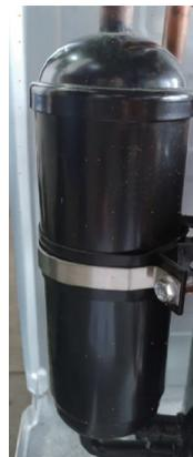
The Accumulator is located in the suction line circuit at the entrance to the compressor. The accumulator helps prevent liquid refrigerant from entering the compressor during run operation.
