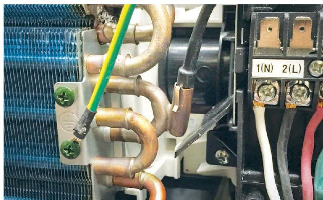
The Piping Temperature Sensor is a negative coefficient thermistor that will decrease in resistance with increases in coil temperature. The sensor is located in a socket soldered to the surface of the indoor coil.
