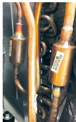
The system has debris-catching strainers that protect internal system components from contaminants in the refrigerant. The strainer is a permanent part that is not typically replaced.
