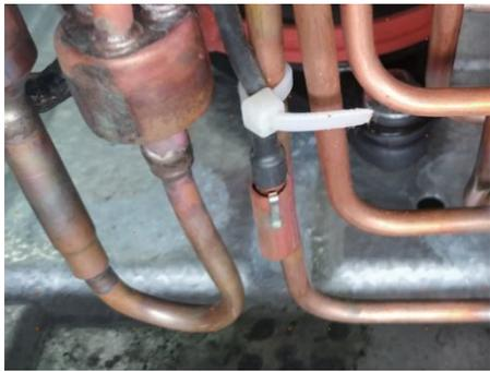
The Defrost Temperature Sensor A is a negative coefficient thermistor that will change resistance in response to outdoor coil temperature changes. The PCB monitors the temperature of the outdoor coil to determine when the system should perform a defrost cycle. The sensor also monitors coil temperature during defrost cycles to determine termination conditions.
