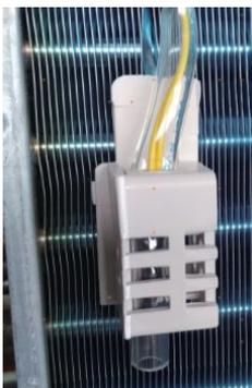
The Ambient Temperature Sensor is a negative coefficient thermistor that will change resistance in response to outdoor air temperature changes. The PCB monitors the temperature of the outdoor air to determine fan speed requirements and inverter speed. The sensor also plays a role in calculation of required defrost conditions.
