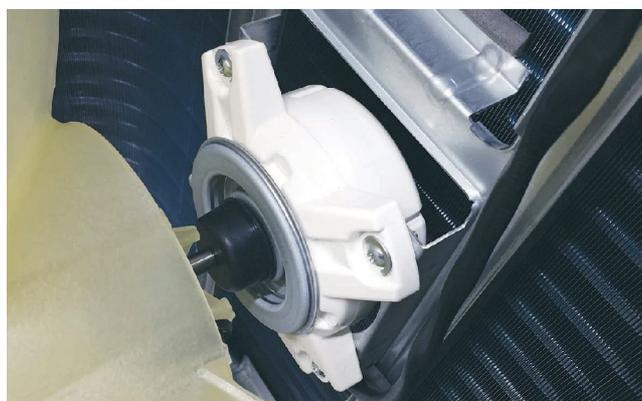
The fan motor is a variable speed motor. The required speed is calculated by the PCB. The motor is electrically connected to the PCB via PLUG CN-21.
