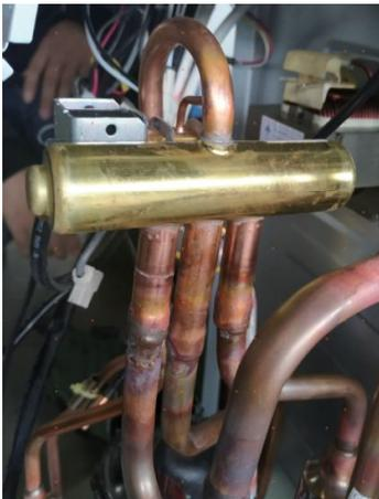
The 4-Way Valve redirects the flow of refrigerant in the piping circuit to allow the system to reverse the functions of the indoor and outdoor coils. When de-energized in COOL MODE, the valve will direct the refrigerant hot gas to the outdoor coil. When energized in HEAT MODE, the valve will direct the hot gas to the indoor coil.
