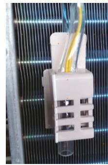
The Ambient Temperature Sensor is a negative coefficient thermistor that will change resistance in response to outdoor air temperature changes. The PCB monitors the temperature of the outdoor air to determine fan speed requirements and inverter speed. The sensor also plays a role in calculation of required defrost conditions.
