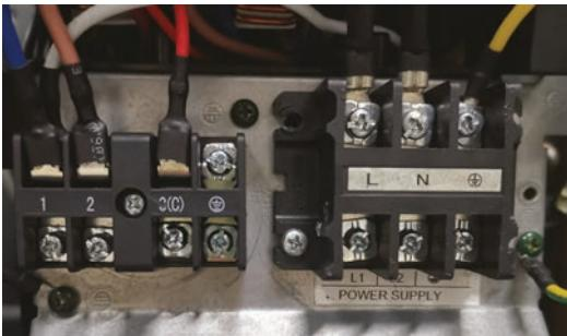
The outdoor unit is powered by 208/230 volt single phase electricity connected at the terminal block. Terminals 1 L (L1) and 2 N (L2) connect this voltage to the system.
