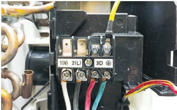
The unit terminal block receives electrical power from the outdoor unit. There are 4 connections for electrical wires. Terminals 1 and 2 are connected to terminals 1 and 2 of the outdoor unit. This wiring supplies power to the indoor unit.
