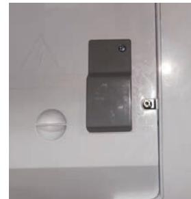
If the remote control is non-functional, the Emergency Button can be used. 73F -78F degrees will be maintained, until commands are received via the remote control.
