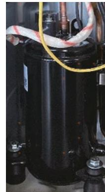
The compressor is a three phase DC inverter driven rotary type, capable of variable speed operation. The compressor operating frequency will be determined by the temperature difference between set point and room temperature.
