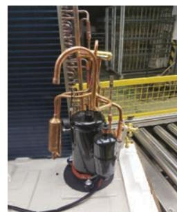
The oil separator is integrated on the exhaust pipe. When the compressor oil passes through the exhaust pipe, it is separated by the oil separator, then returns to the air return pipe through the oil return capillary, and then returns to the compressor.
