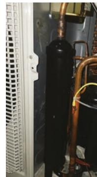
The liquid and gas separator is located on the suction line circuit before accumulator. It can help prevent the liquid refrigerant entering the compressor during the operation.
