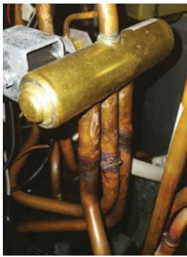
The 4-Way Valve redirects the flow of refrigerant in the piping circuit to allow the system to reverse the functions of the indoor and outdoor coils. When de-energized in COOL MODE, the valve will direct the refrigerant hot gas to the outdoor coil. When energized in HEAT MODE, the valve will direct the hot gas to the indoor coil.
