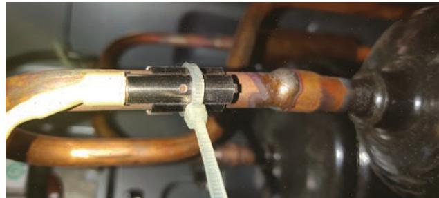
The Suction Line Temperature Sensor is a negative coefficient thermistor that senses the temperature of the suction line. The PCB monitors the temperature of the suction line and the EEV operation to maintain an acceptable superheat.
