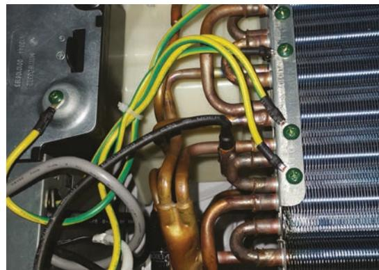
The Piping Temperature Sensor is a negative coefficient thermistor that will decrease in resistance with increases in coil temperature. The sensor is located in a socket soldered to the surface of the indoor coil.
