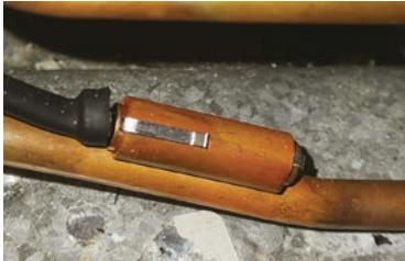
The Defrost Temperature Sensor A is a negative coefficient thermistor that will change resistance in response to outdoor coil temperature changes. The PCB monitors the temperature of the outdoor coil to determine when the system should perform a defrost cycle. The sensor also monitors coil temperature during defrost cycles to determine termination conditions.
