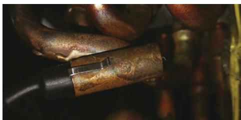
The Defrost Temperature Sensor B is a negative coefficient thermistor that will change resistance in response to outdoor coil temperature changes. The PCB monitors the temperature of the outdoor coil to determine when the system should perform a defrost cycle. The sensor also monitors coil temperature during defrost cycles to determine termination conditions.
